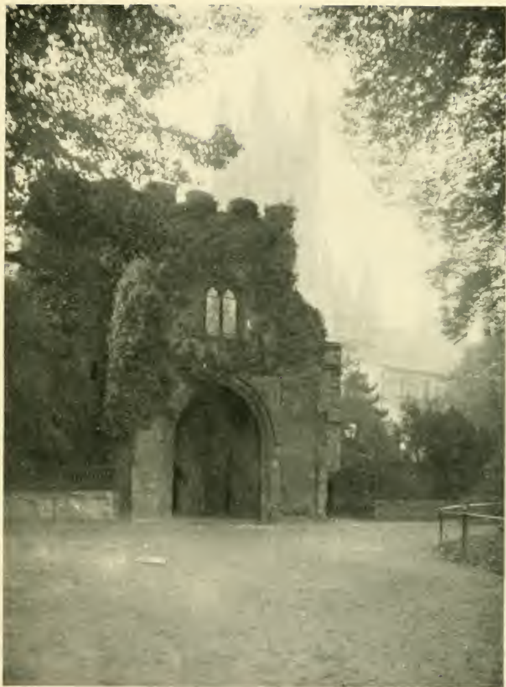
CANTERBURY CATHEDRAL, AND PART OF MONASTIC BUILDINGS, FROM PRIOR'S GREEN.
